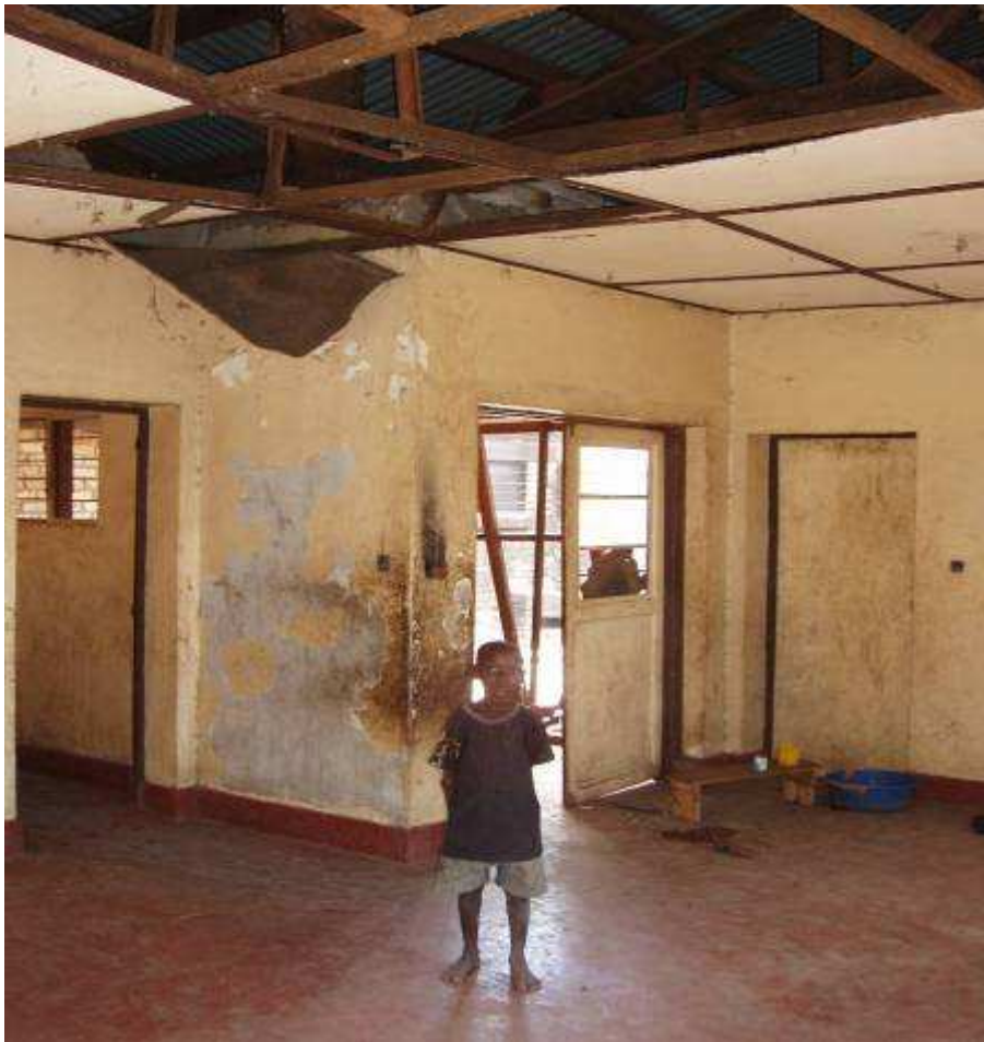
Before HIV renovation work October 2006
