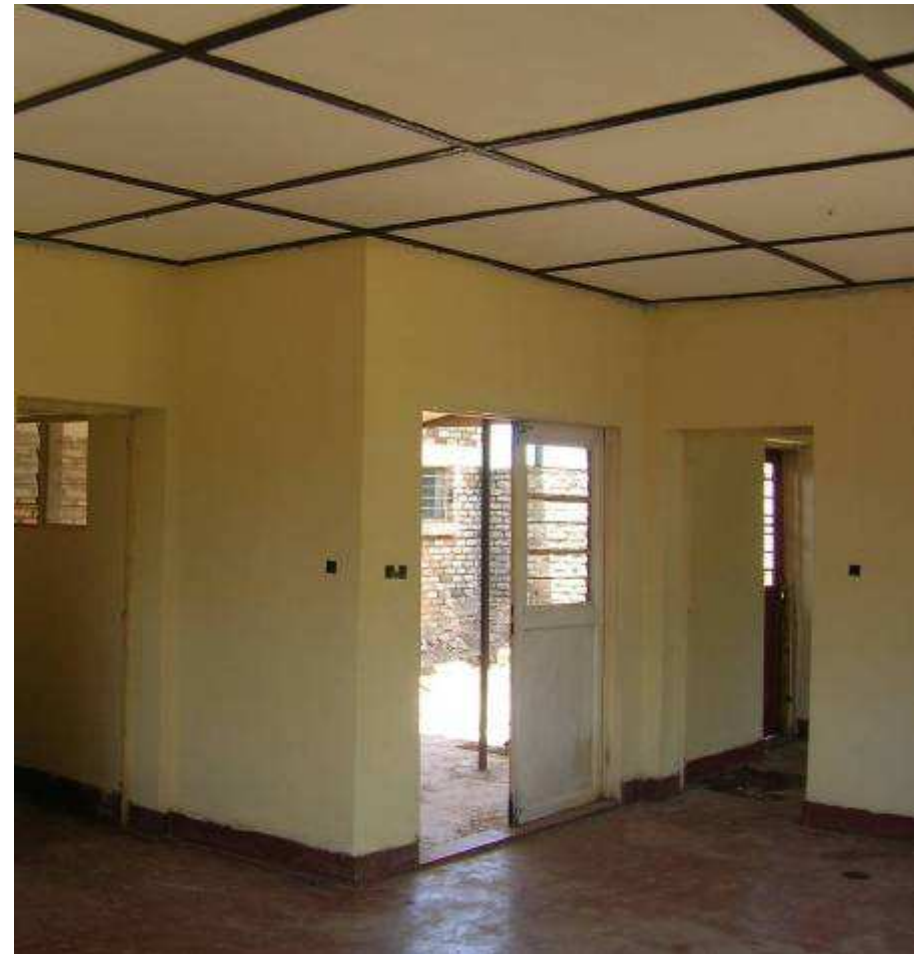
Renovations still in progress: February 2007
