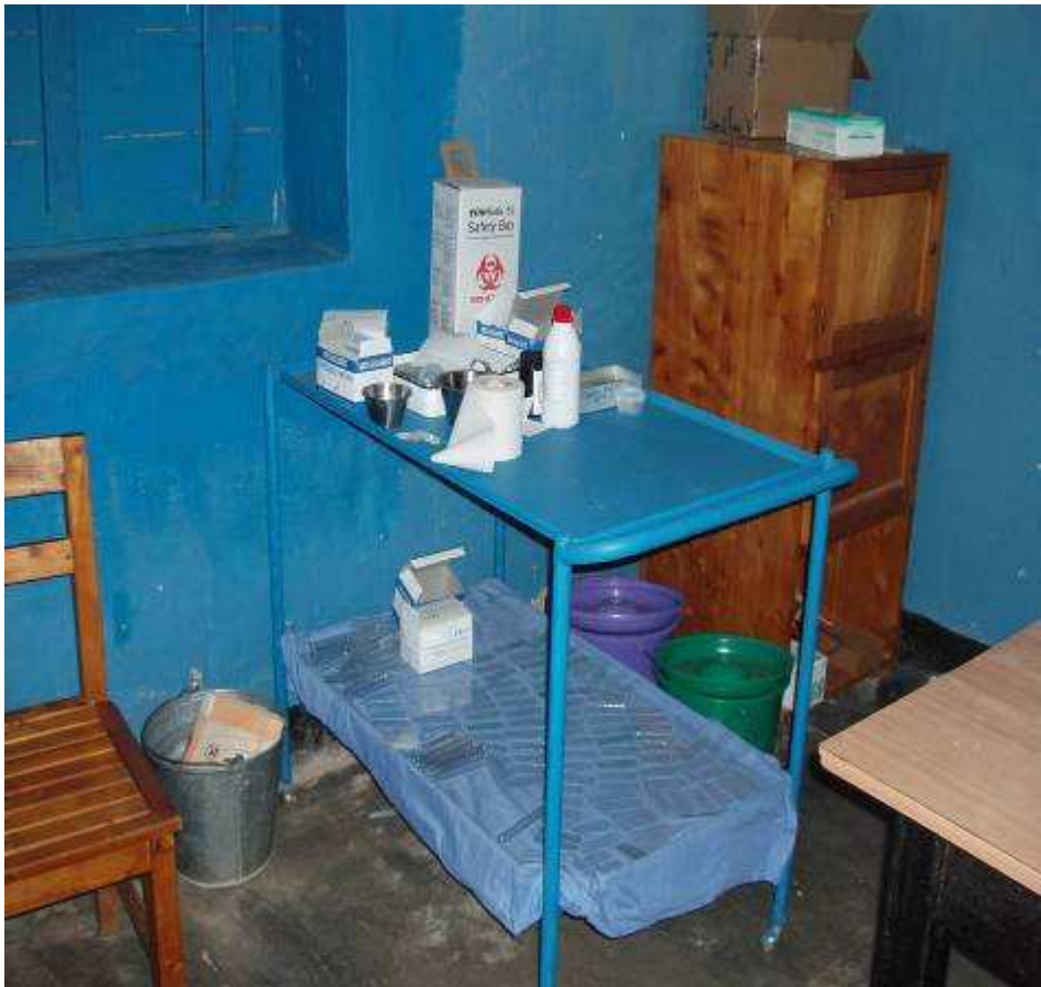
Before HIV renovation work
